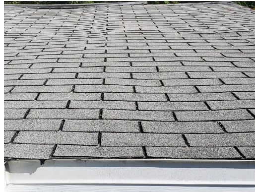
1941-1 Asphalt Shingle/Tar Typical Exterior Roof
